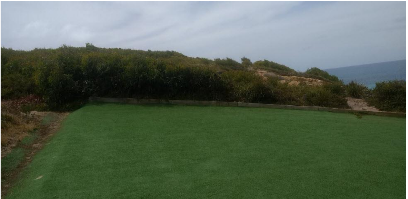
4 East side of launch with spoon drain
